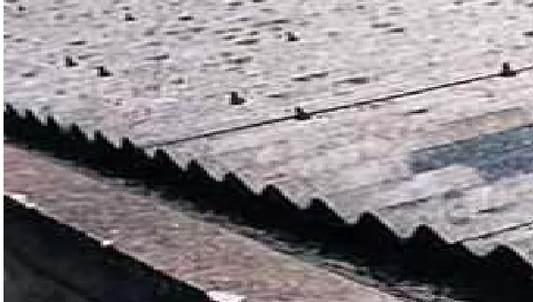
Fig 8: Asbestos Cement Roof Sheeting & Gutters.
