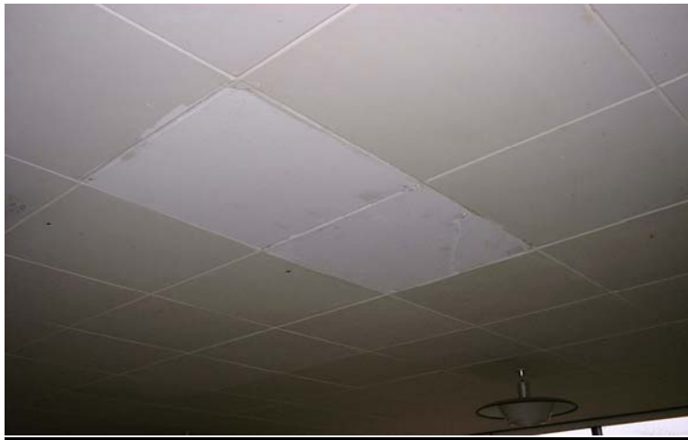
Fig 6: Asbestos Containing Ceiling Panels.
